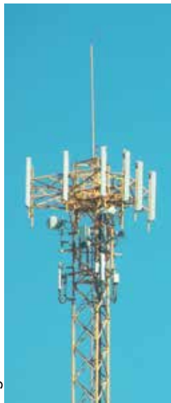
Figure 1: Cell site with three sectors
